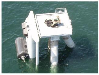
14 each of 6 ft diameter x 16 ft **long Ocean Guard™** Netless foam filled fenders with integral swivel end fittings.
